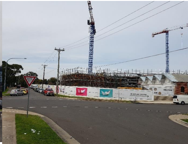
Figure 10 – View of the Paper Mill development currently under construction, located directly opposite the site.
